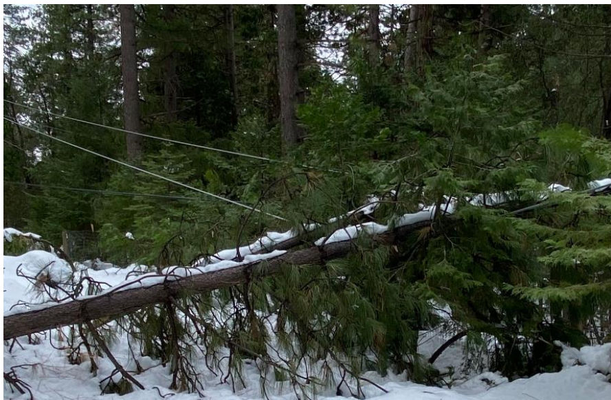
FIGURE PG&E-22-11-3: COVERED CONDUCTOR EFFECTIVENESS – EXAMPLE 3
